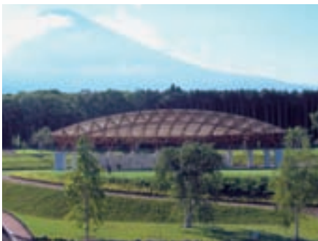
■ Gotemba Fuji Exchange Facility Location: Shizuoka
