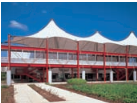
■ Inzai Elementary School Location: Chiba
