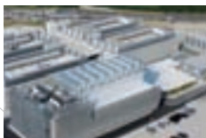
Data Center with Transferred Server
